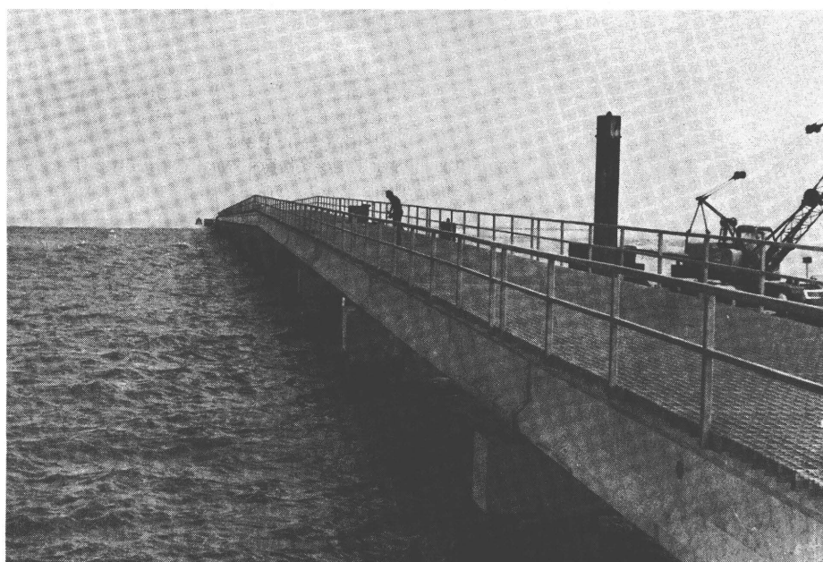
Causeway for the new deep water port in Belize city: the 1980 agreement provided for closer cooperation between Guatemala and Belize in the area of transport
