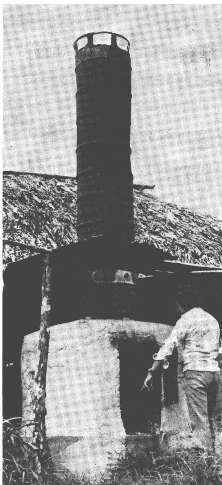
A corn and peanut drier (above) was built using local materials on Tzib's farm in San Antonio, Belize—and a simple peanut sheller has been introduced and is very popular with farmers
