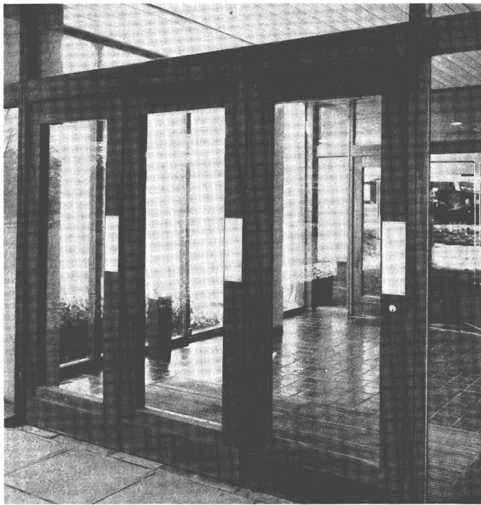
Tropical hardwood is often used for high-class joinery, as in these entrance doors to a public building
