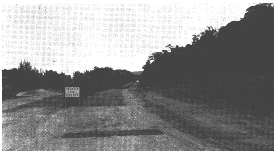
Road maintenance in North Efate.
