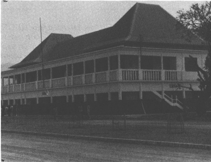
Eséka station was built by the Germans before 1914, extended in 1925 and modernized as part of the realignment operation
