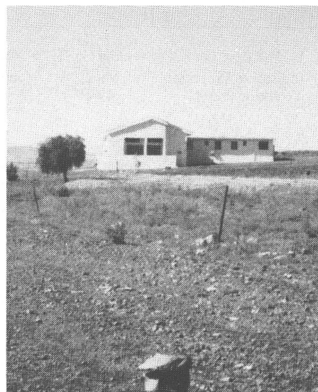
Post office at Bataung, one of 18 built with EDF assistance
