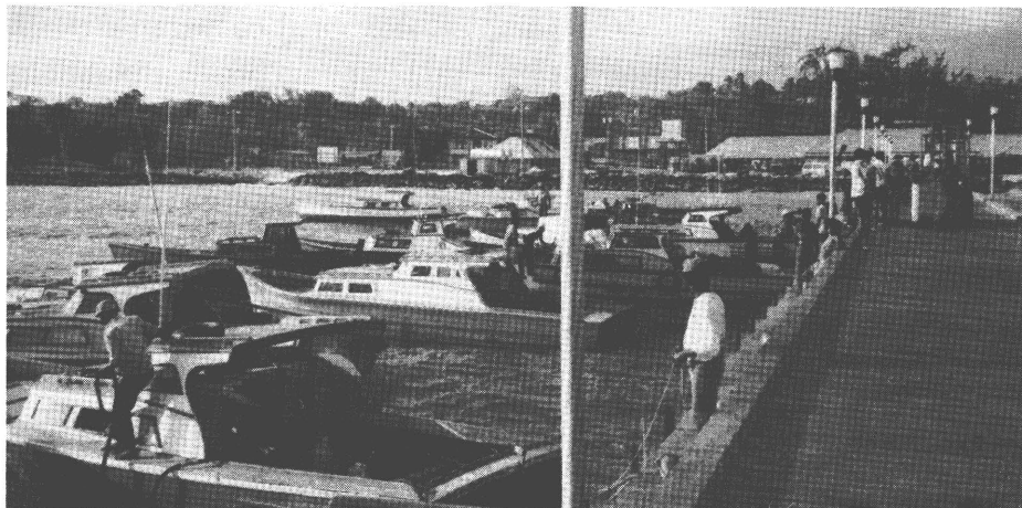
The Oistins Fisheries Complex, an integrated fisheries landing, processing and marketing facility, benefiting fishermen, vendors and the buying public alike (Lomé I Indicative Programme)
