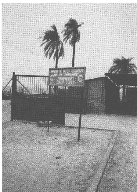
The fisheries station at Gunjur where much of the infrastructure for the artisanal fisheries project is situated
