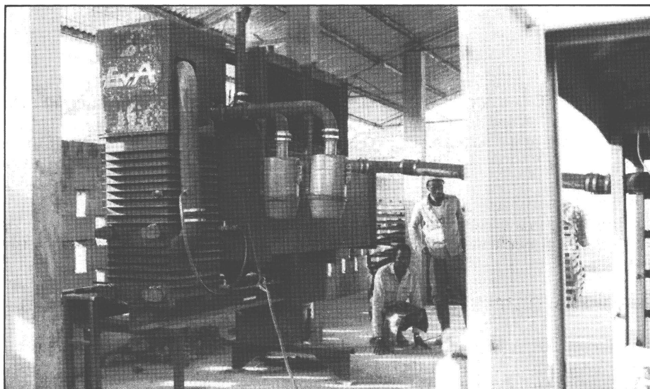
This fixed version of the gas generator was installed with CID assistance in the Gambia.
