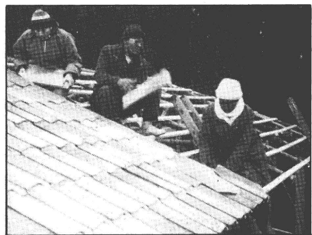
A small roof-tile production unit and the laying of the tiles on a roof.
