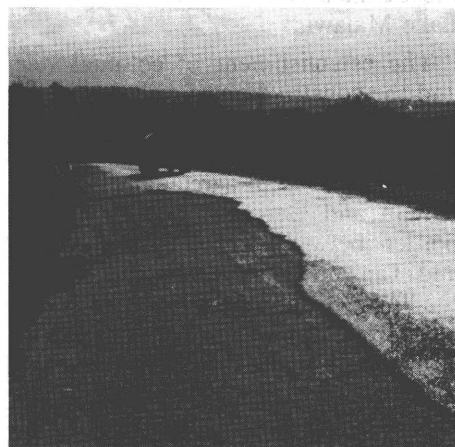
Some stretches are in an advanced state of disrepair
