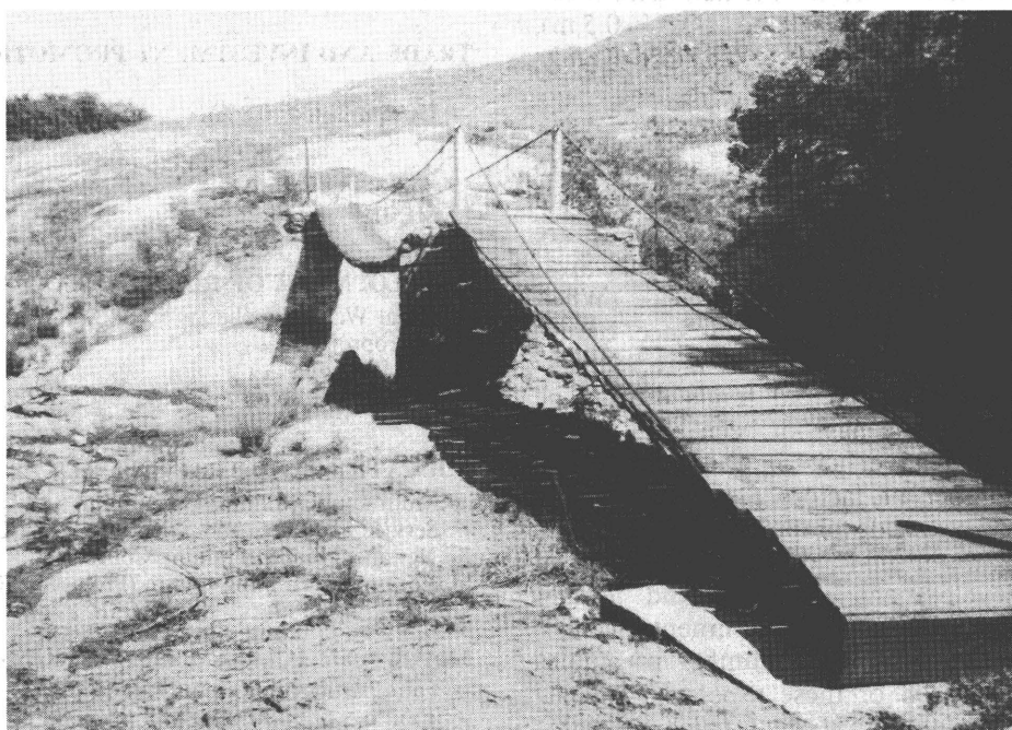
The footbridge across the Lusushwana river
