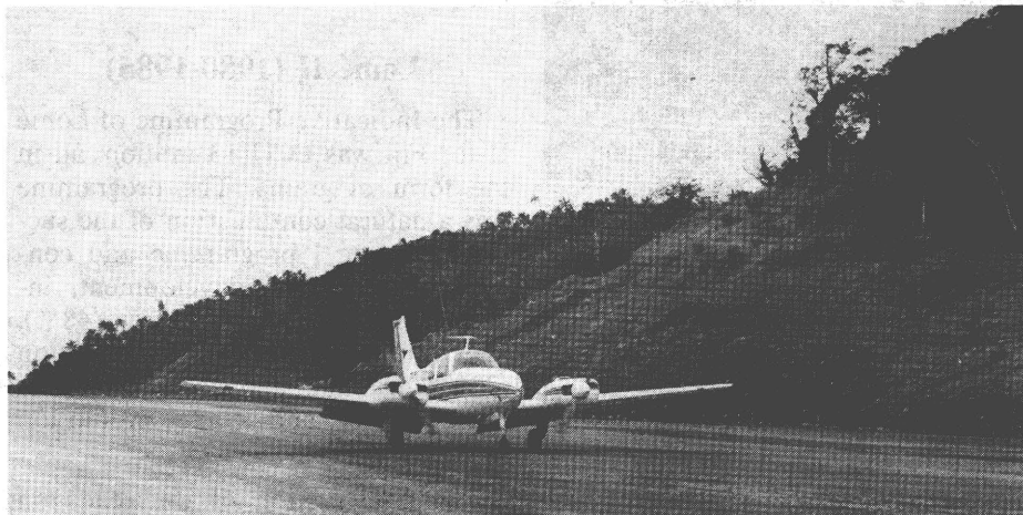
The construction of airstrips on three Outer Islands (above Moala) contributed towards the economic, social and administrative integration of Fiji
