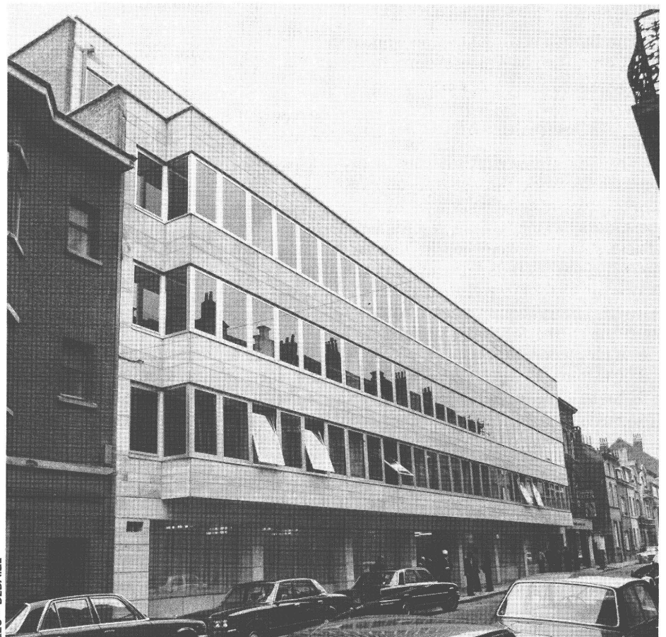
ACP House in Brussels
