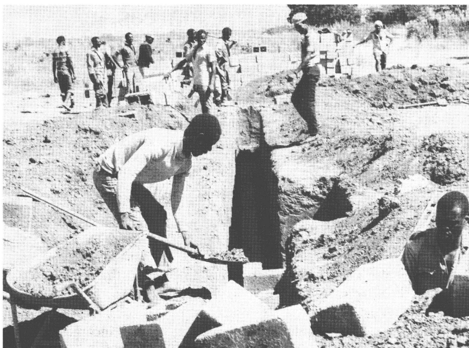
Laying foundations made of stabilized laterite
