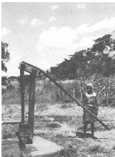
An EEC borehole with pump near Nizmazuwa. Such pumps are highly valued by the village community, in particular by women, as they considerably lighten their workload
