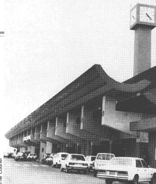
The EDF has contributed significantly to the rehabilitation of the Transcameroon railway for which a new station has been built in Douala (above)
