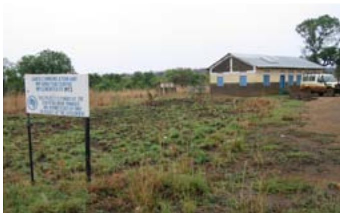
Photo 5 — A communication and information centre for the 'Sudan community-based recovery and rehabilitation programme (RRP)'
