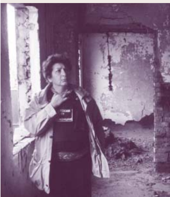
Costanza Adinolfi inspects a war-damaged building in Chechnya.
