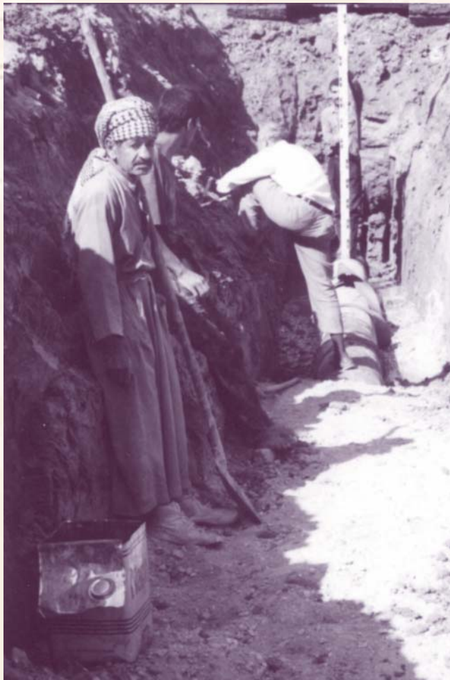
New pipes to ensure a supply of clean drinking water.
