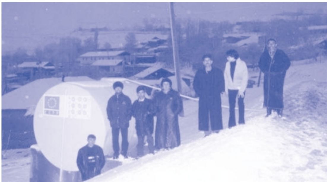
VILLAGERS OF SAVLA IN FRONT OF THEIR NEW WATER TANK.
