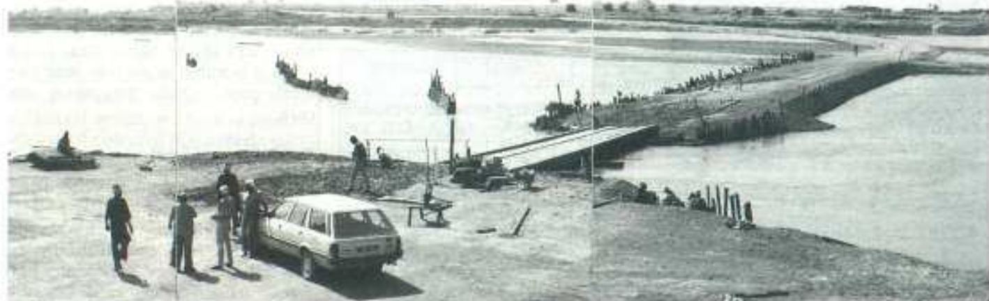
Using this temporary bridge, financed by the EEC, 75 000 t of emergency food aid and 25 000 t of petrol have transited to Chad
