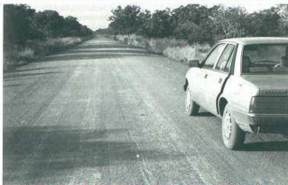
This road linking N'Djamena to Sarh in the South is currently being rehabilitated with EDF financing
