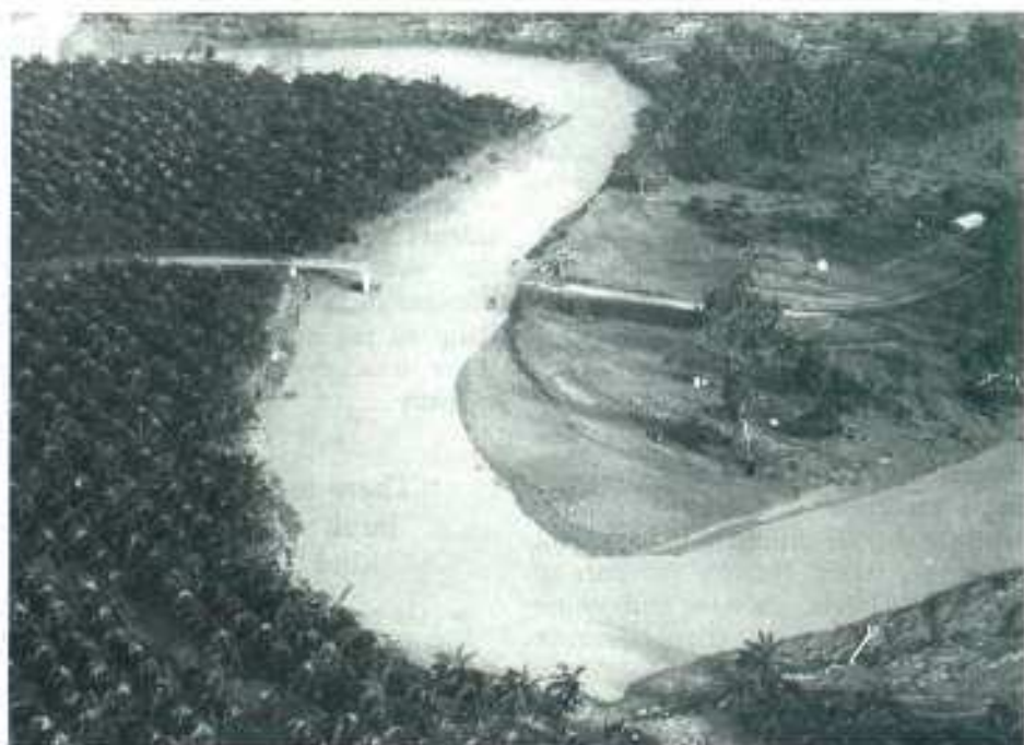
Destruction of Vouza Bridge on Guadalcanal. This was repeated on a massive scale
