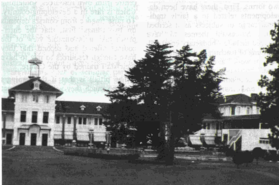
General view of the Hôtel des Thermes at Antsirabe
