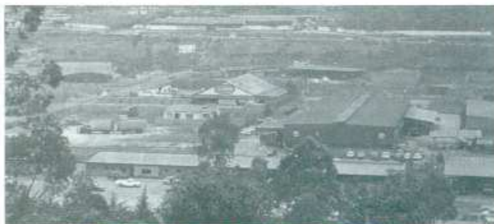
The Kigali Industrial Estate, built with EDF funds
