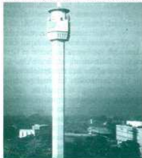
TV transmitter at Bouaké (C.I.)
