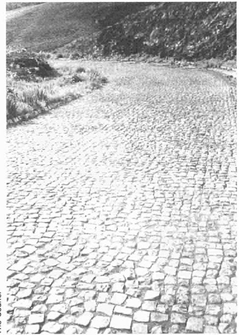
Paving roads, a technique the Cape Verdeans are perfectly accustomed to
