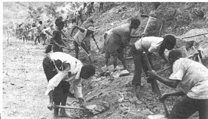
A labour-intensive road construction project in Burundi
