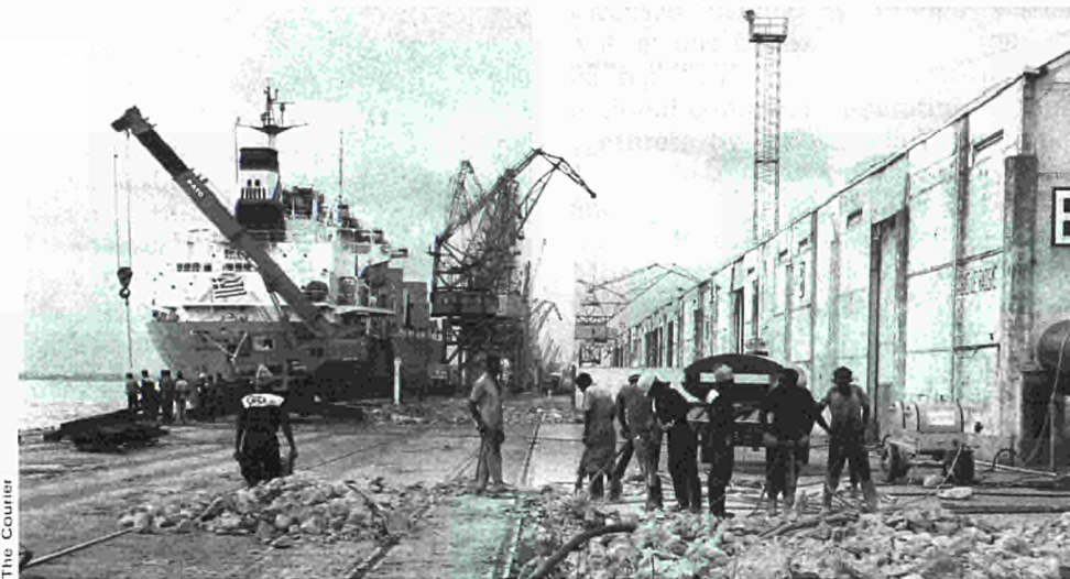
Rehabilitating Maputo Port — the first crane will also be overhauled
