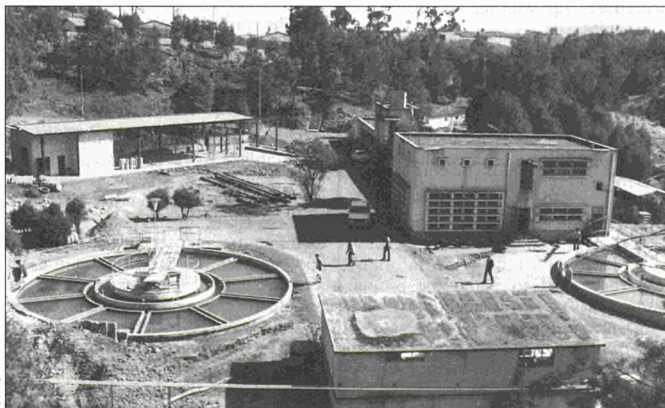
Extension work on the treatment plant at Gafarsa
