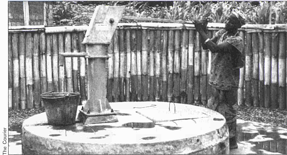
A water pump caretaker in one of the villages demonstrating how it works
