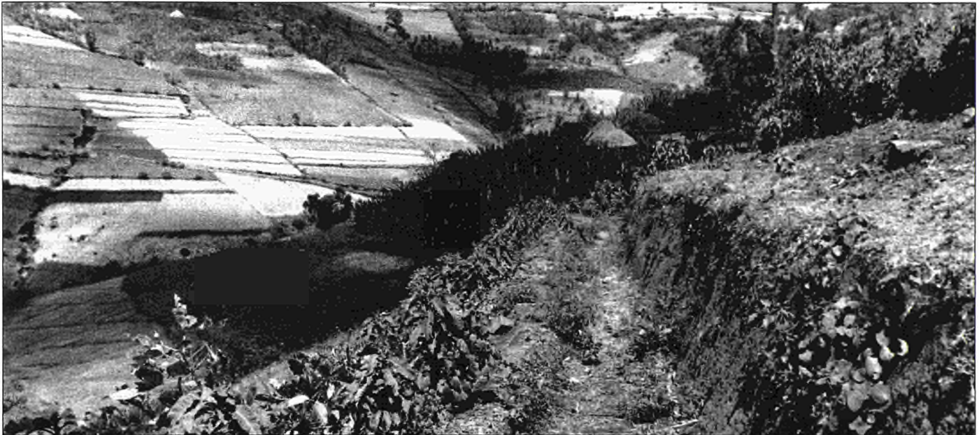
A cut-off drain in South Shewa — one of a number of techniques that help to check the formidable erosive power of run-off water
