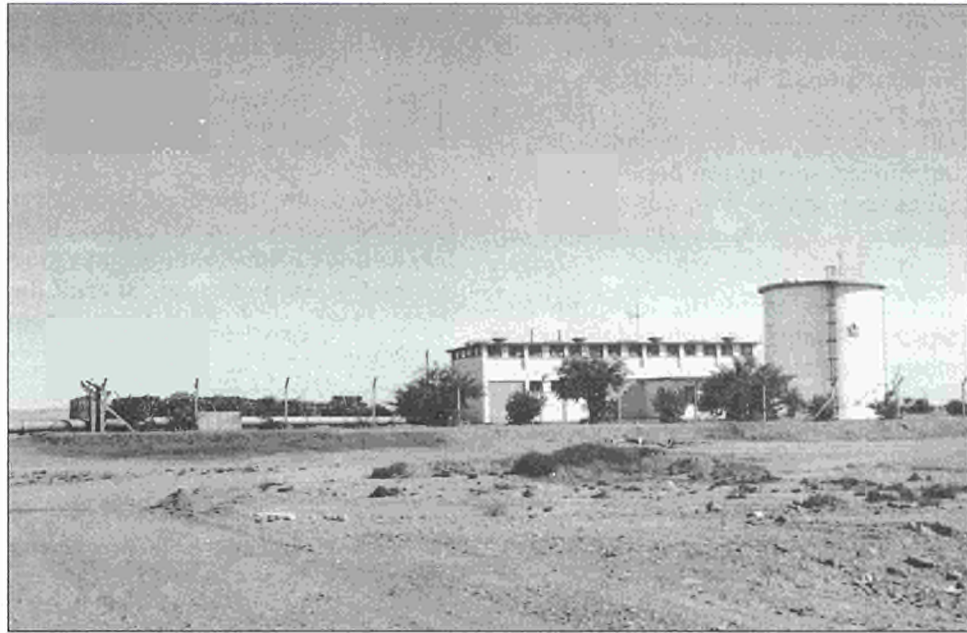
A water pumping station in the Namib desert
