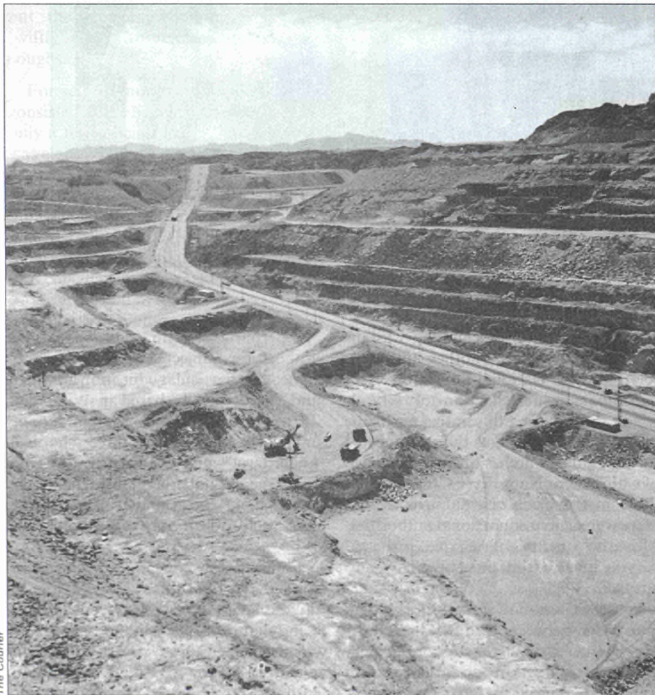
A view of the 'pit'
