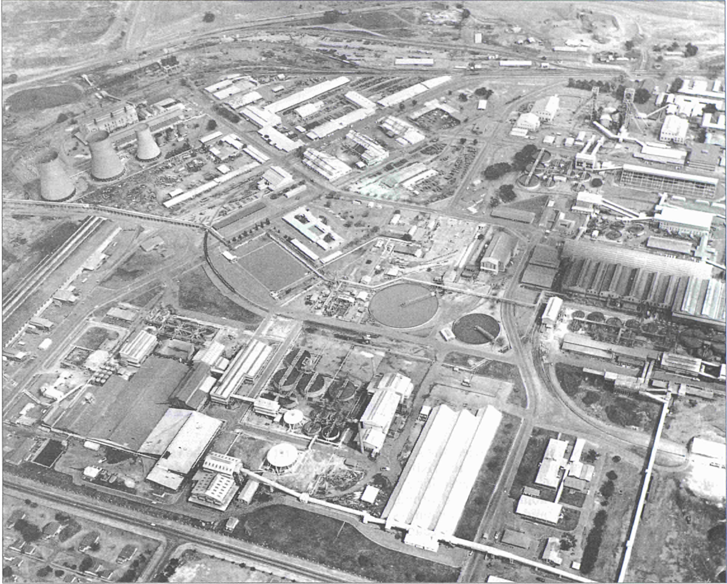
General view of the copper plant area at Nchanga (Zambia)
