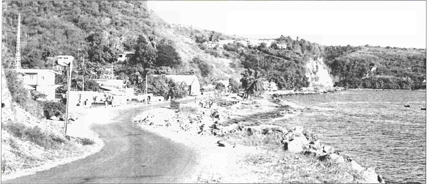
This EDF-financed coastal road near Salisbury was resurfaced and provided with sea defences after Hurricane David
