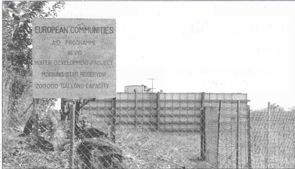
Considerable efforts were made to improve the water supply system on Nevis
