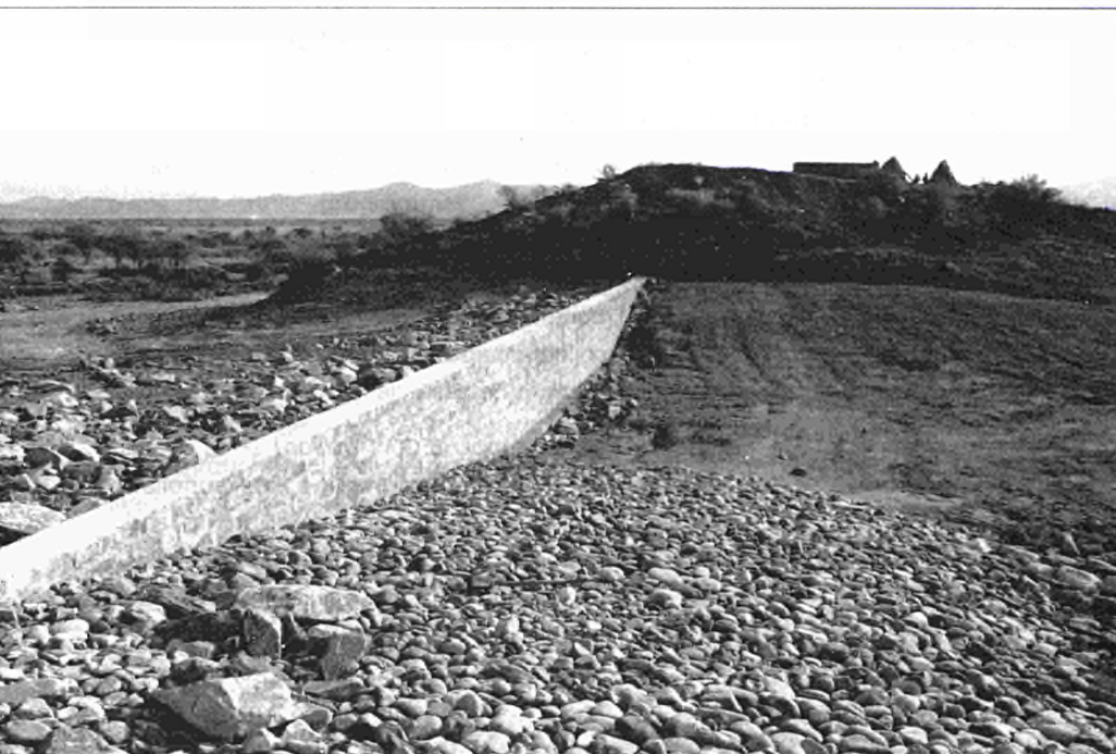
Small-scale dams like this one in the highlands will trap water for irrigation
