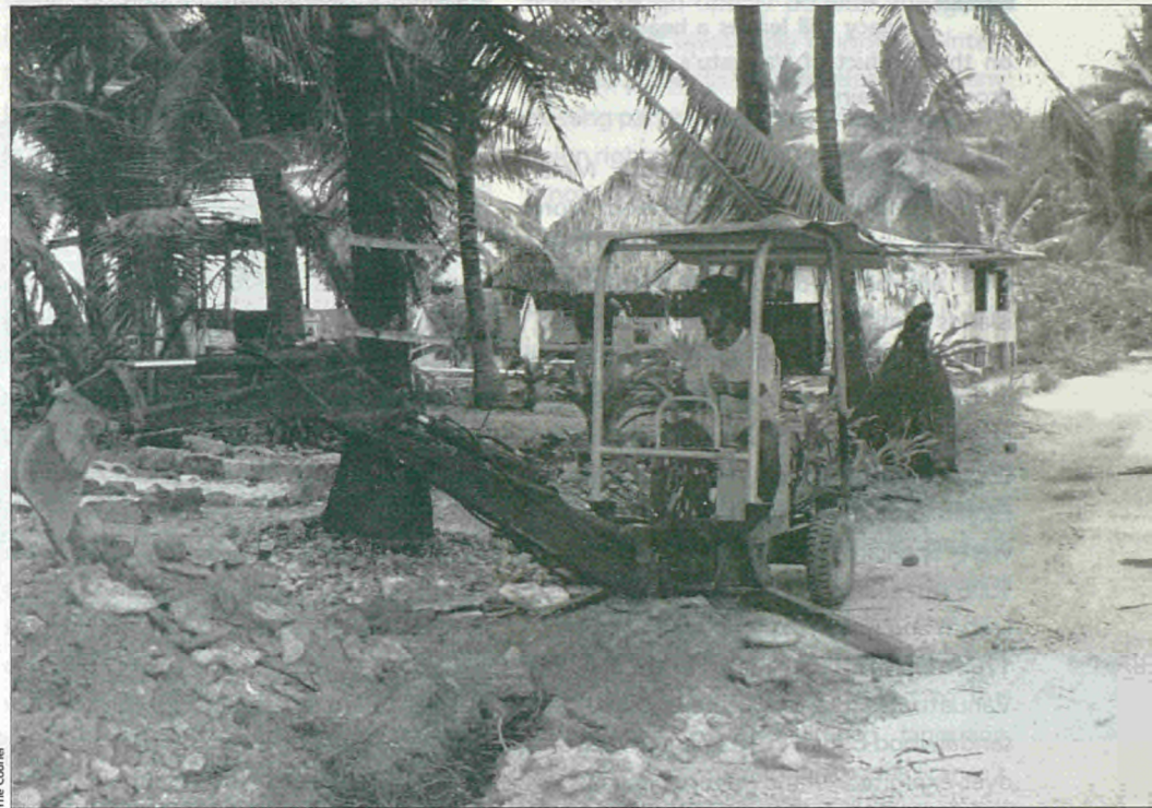
Laying cables to expand the electricity distribution network on Funafuti — using Lomé funds
