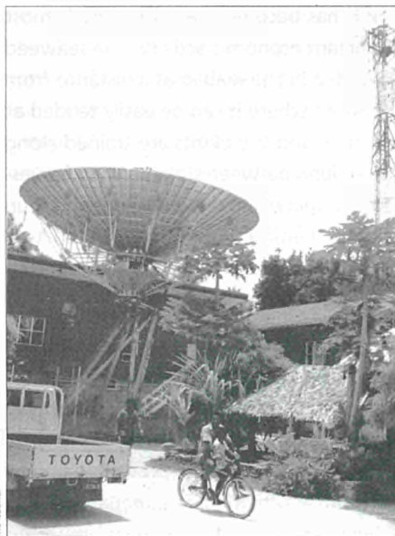
The satellite ground dish and telecommunications mast which link Kiribati's capital Tarawa to the outer islands and the world. EU aid to Kiribati has focused on this sector
