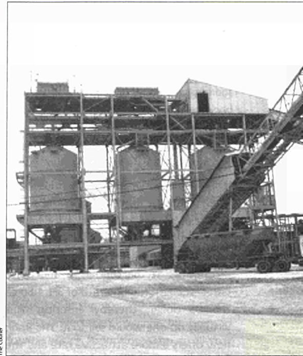
Part of Suralco's bauxite processing plant at Paranam near Paramaribo
