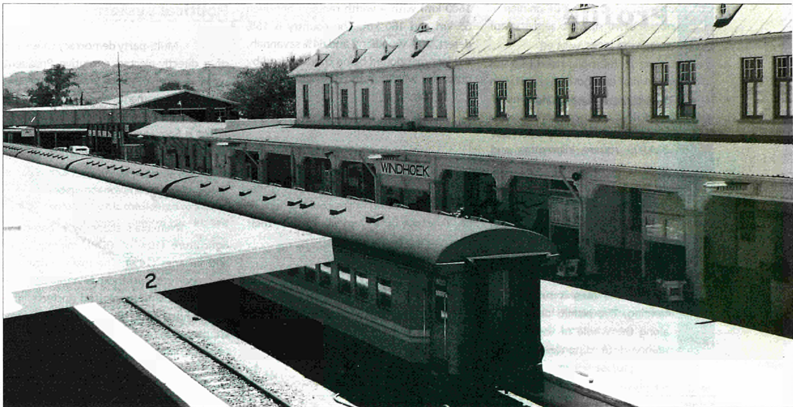
Windhoek Railway Station 'We have up-to-date infrastructures which are among the best on the African continent'
