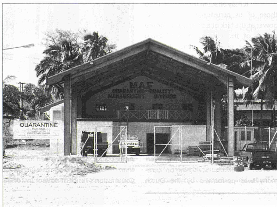
The new quarantine building at Neiafu
