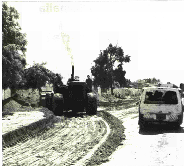
Road repairs in Mogadishu organised by a private entrepreneur
