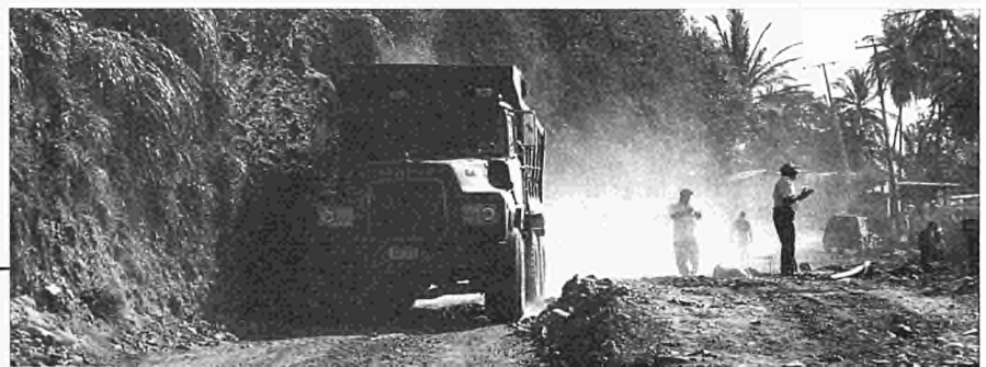
Road rehabilitation in progress.
