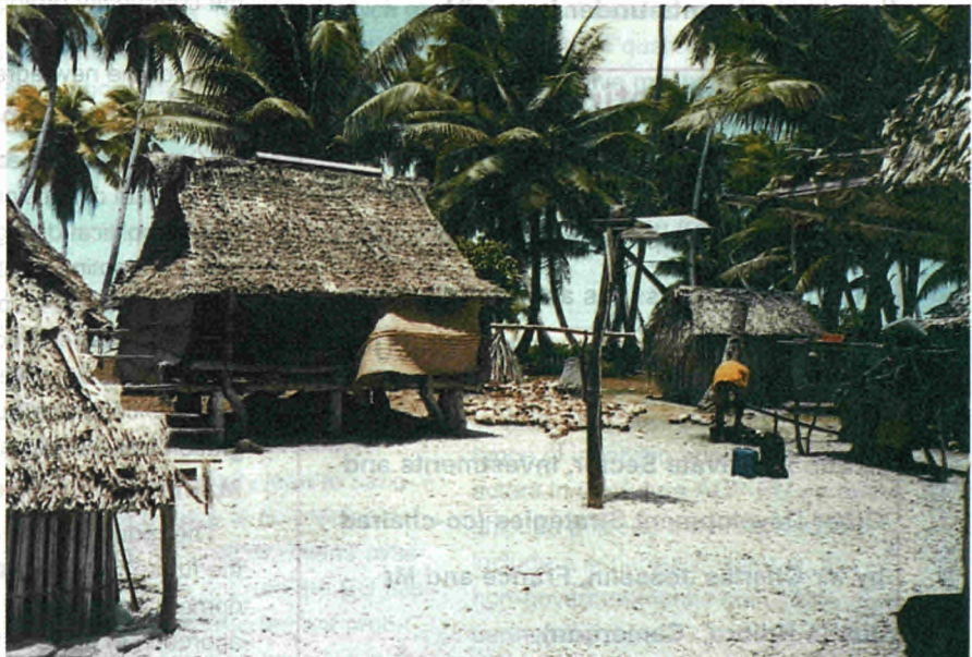
PV panels mounted on the apex of the roof and an outside light on a pedestal
