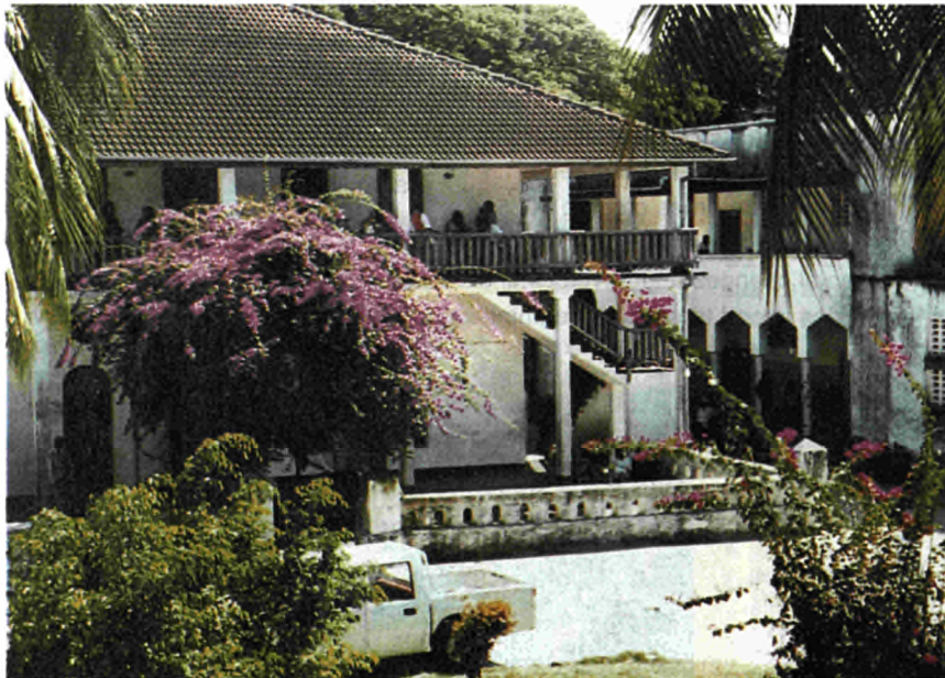
Sea breezes cool the old colonial hospital building
