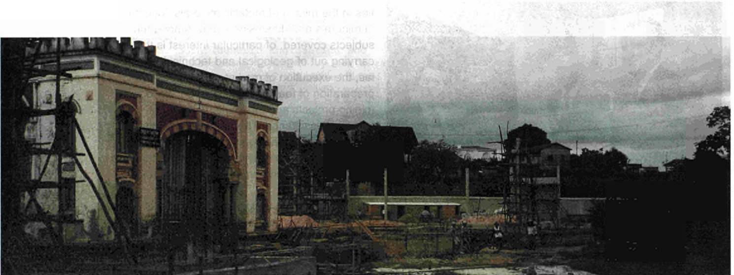
The construction work is in progress
