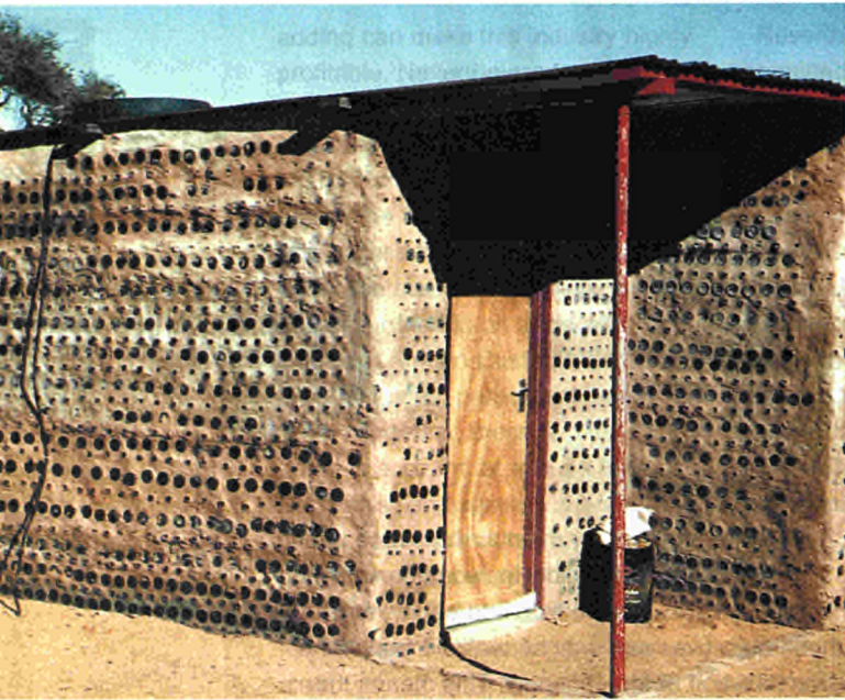
Making the most of what they have. People build houses skillfully with walls of mud and bottles
