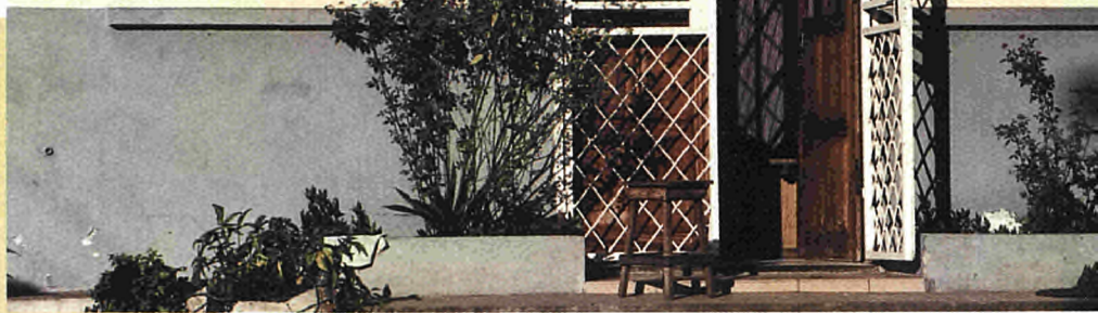
Renovation of a health centre, Brazzaville
