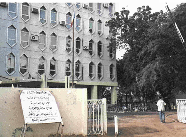
Ministry of Education, a nine-storey building without elevator. In the hottest months (50°C) tea is served halfway up the stairs.
