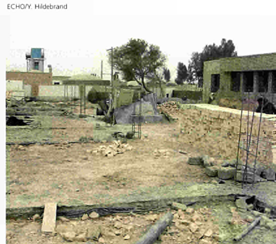
Reconstruction of a hospital in Zaranj - Afghanistan.
