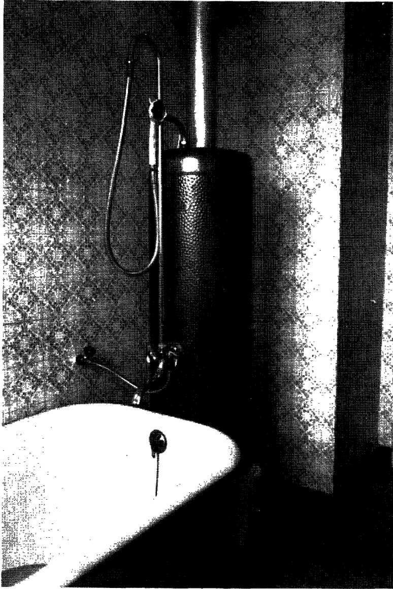
DORTMUND – Sanitary installation before modernization
