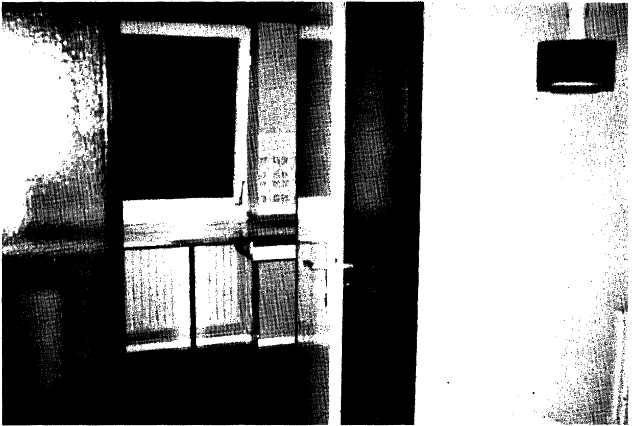
DORTMUND – Translucent prefabricated partition between kitchen and dining space
