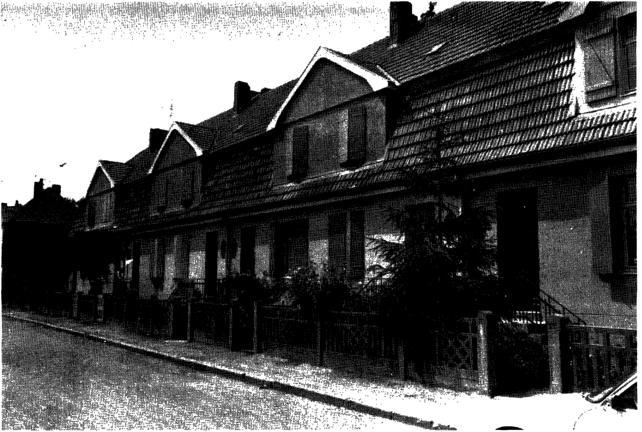
HAGONDANGE – Modernized houses – boundary fences will be progressively raised to the level of plinth walls
