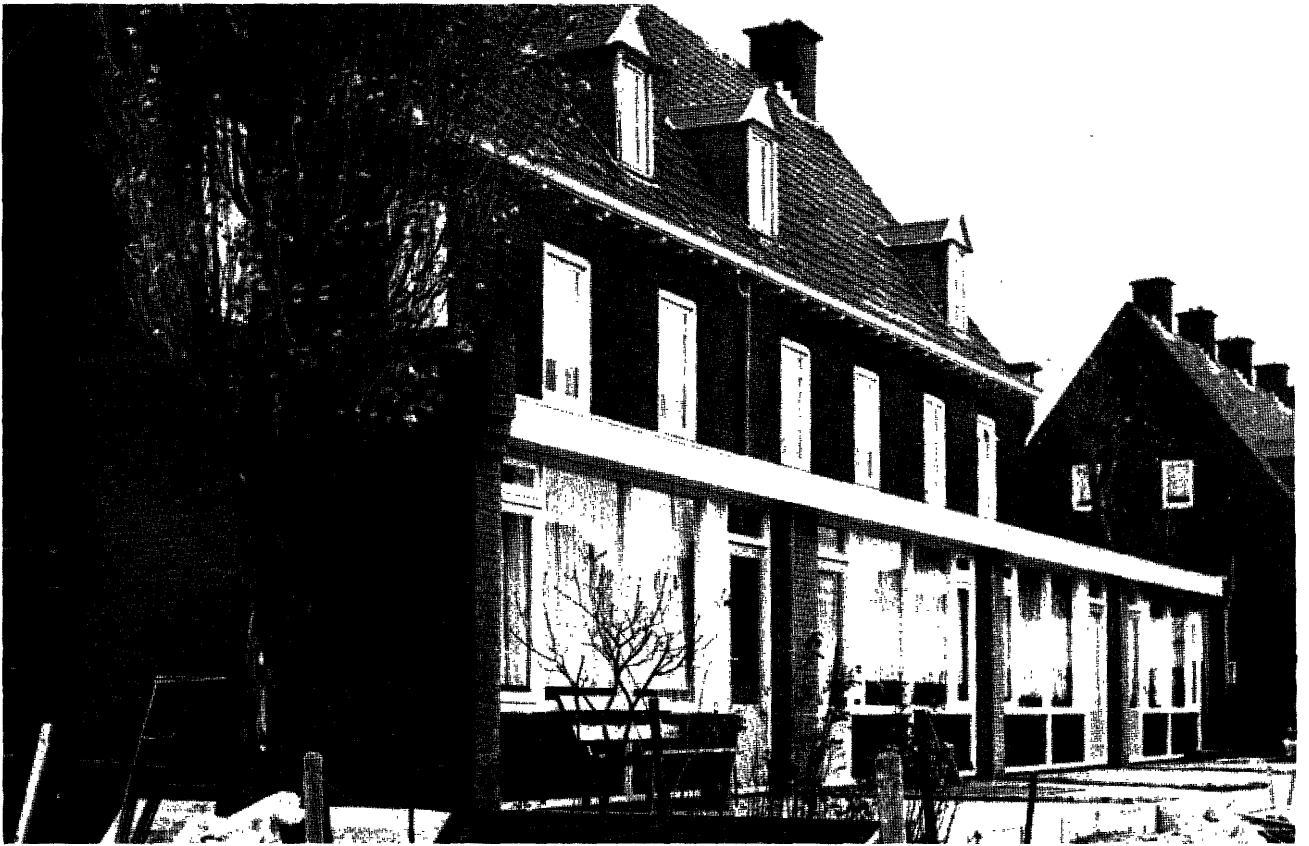
HEERLEN – The new living-rooms with terrace extension (prefabricated facades)
