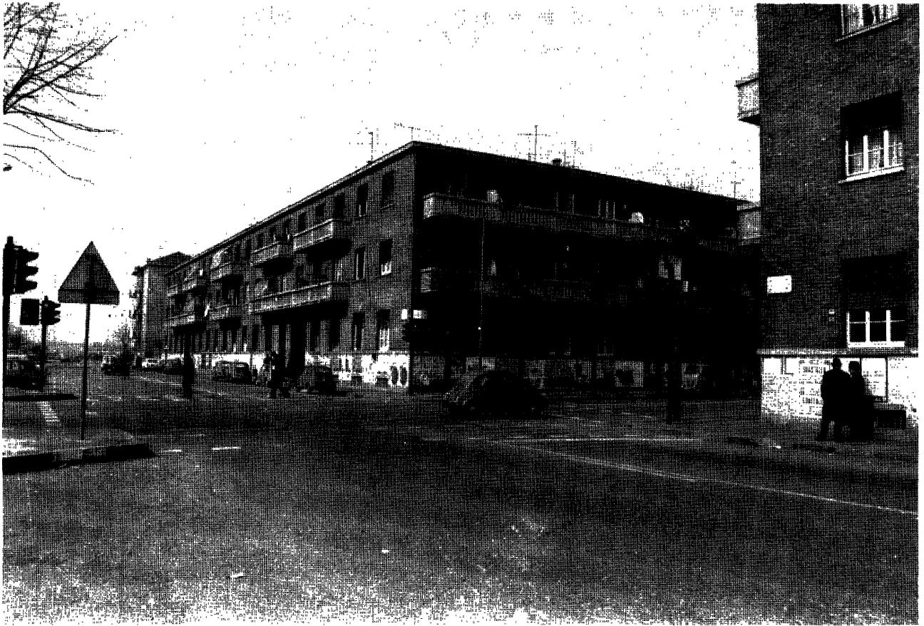
SESTO SAN GIOVANNI – Apartment blocks included in the experimental programme of modernization
