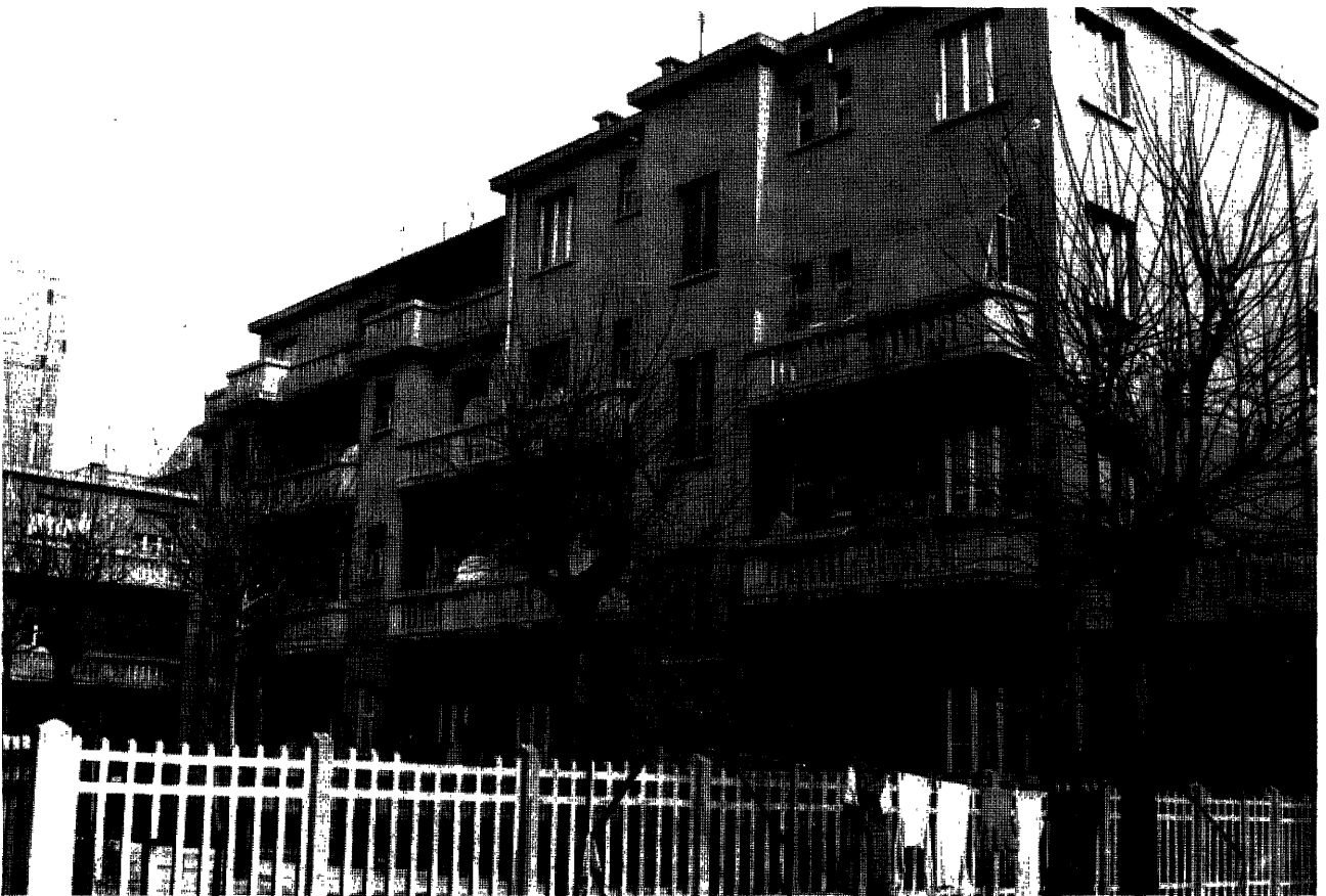
SESTO SAN GIOVANNI – Apartment blocks included in the experimental programme of modernization
