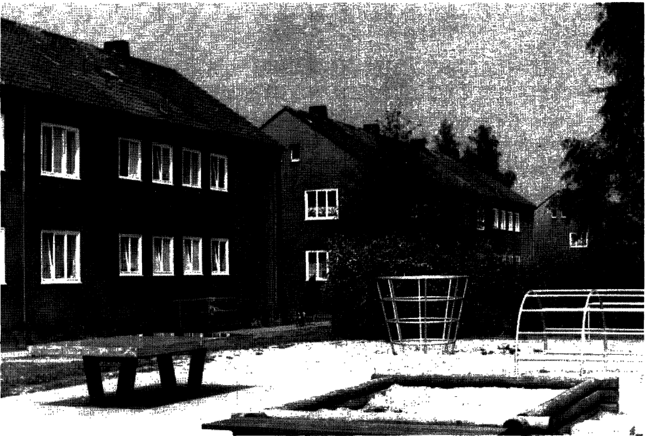
HEESSEN – Improvement of the surroundings – children's play-space
