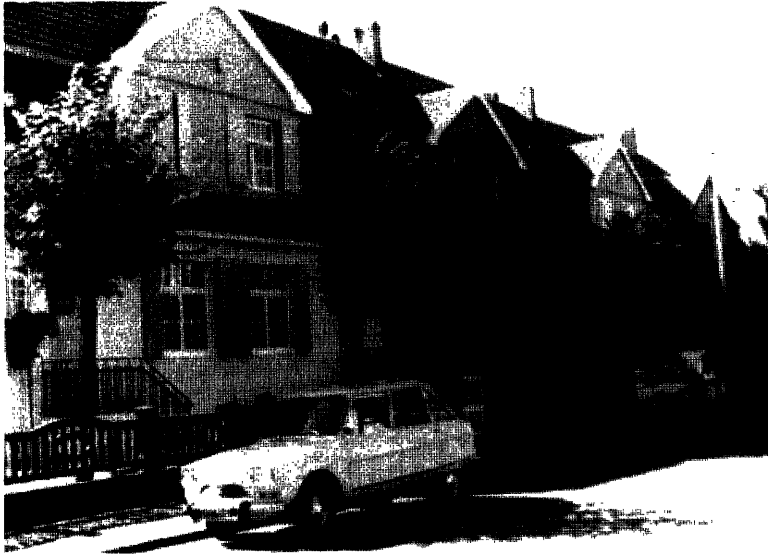
HAGONDANGE – Modernized terraced houses (plastering and external paintwork matched by the colour consultant)
