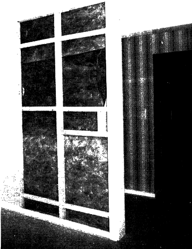
DORTMUND – Prefabricated timber-framed partition walls sandwiched between plasterboard panels
