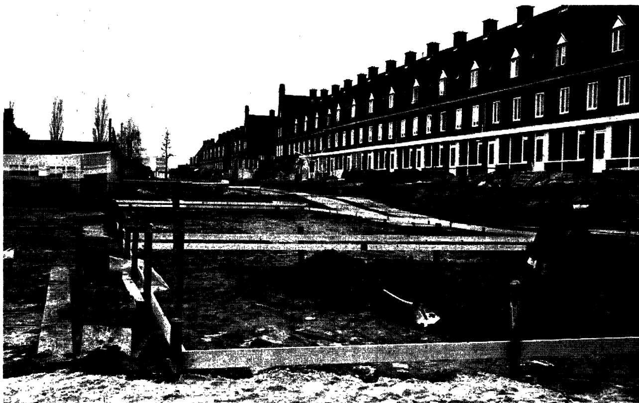
HEERLEN — Foreground: construction of garages — Background: track for crane used in enlarging living rooms and building terraces
