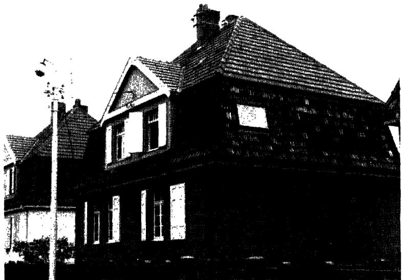
HAGONDANGE – Individual modernized house (note the prefabricated frame which opens, lighting the bedroom)
