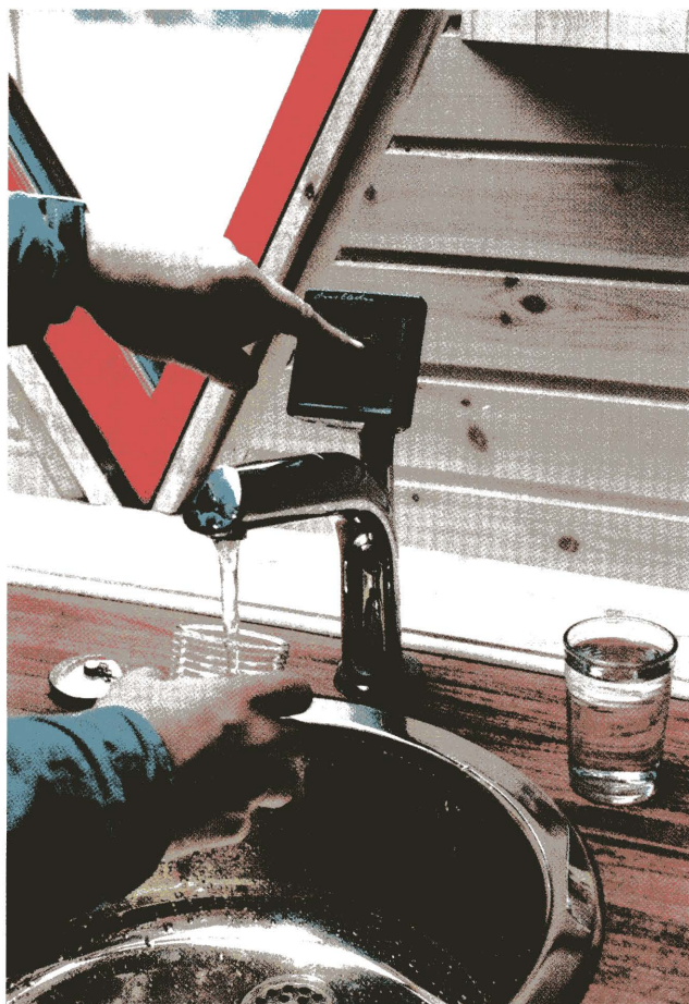
Pict. 8.2 The intelligent tap which can be programmed to give a pre-defined water volume with the right temperature.
