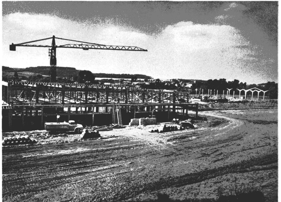
La Cellulose des Ardennes - Building the mill.
