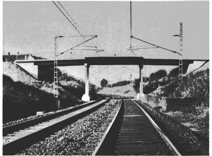
Road bridge at Kerzell after electrification.
