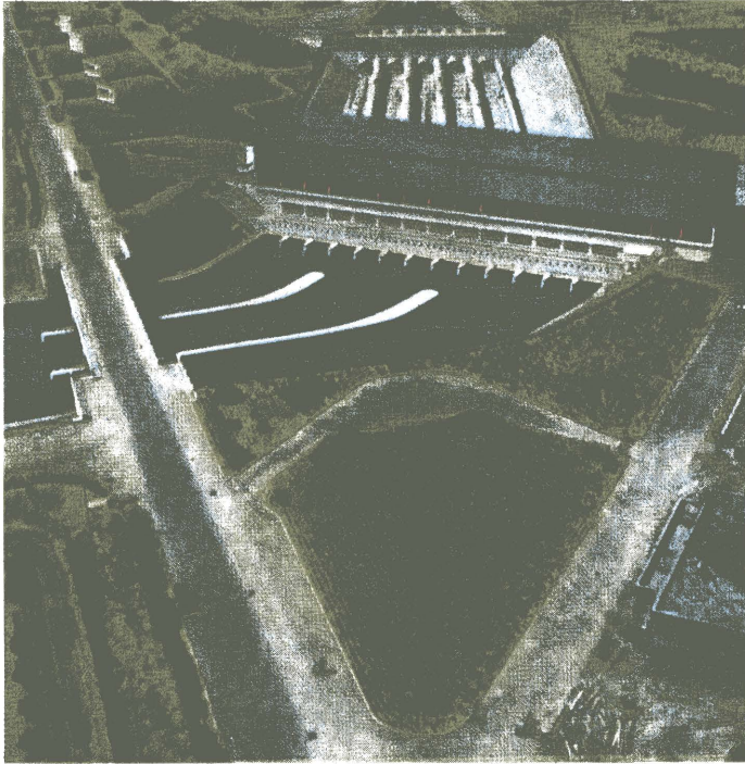
Bas-Rhône Languedoc - The Aristide Dumont pumping station.
