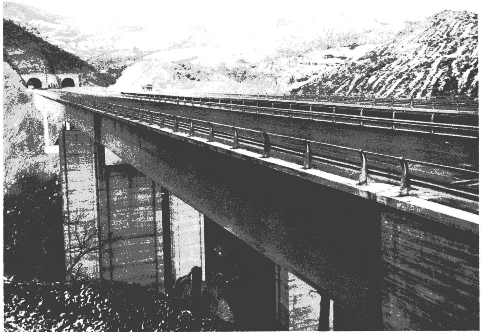
Bridge on the Motorway of the Sun.
