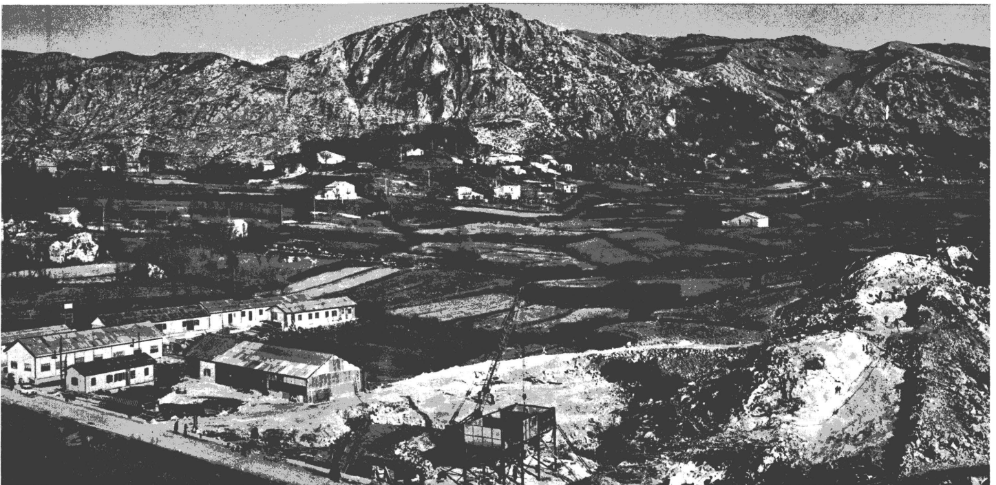
Gallo (Campania) - Dam construction site.
