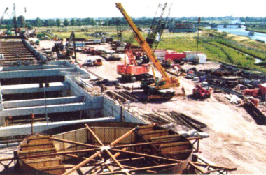
Construction of HSL-Zuid
