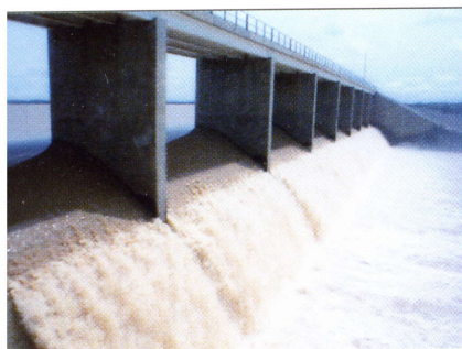
Ziga dam, Burkina Faso
