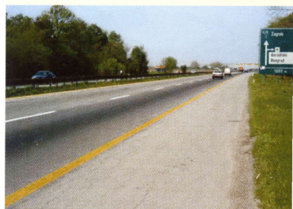
Modernisation of road network in Serbia and Croatia
