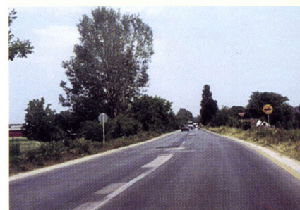
Rehabilitation of roads in Bosnia-Herzegovina
