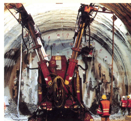
Bologna - Florence high-speed rail line
