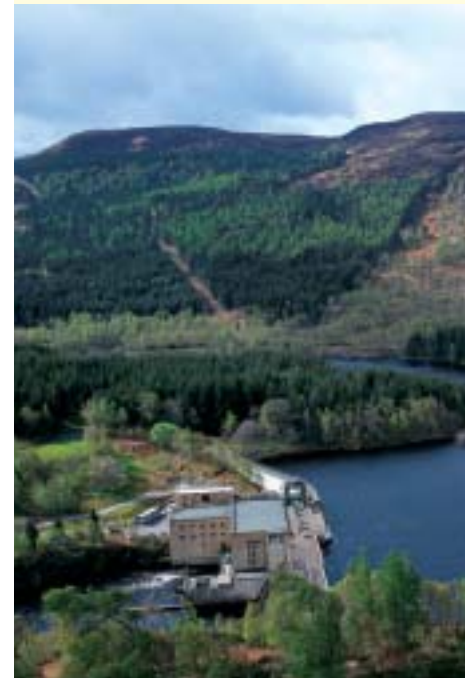
Hydroelectric power plant, Torrachilty (Scotland)
