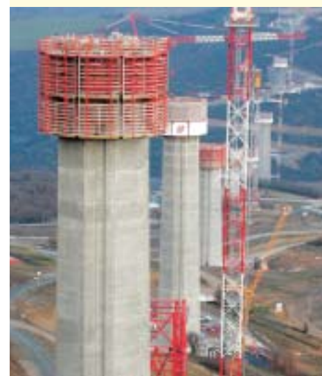
Construction site of Millau bridge, Aveyron
