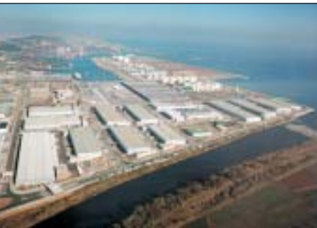
Intermodal terminal, Barcelona
