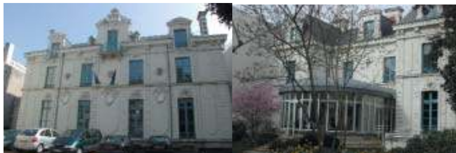
The 'Hotel Bordeaux-Montrieux', premises of the CPVO in Angers (F) (front and back views)
