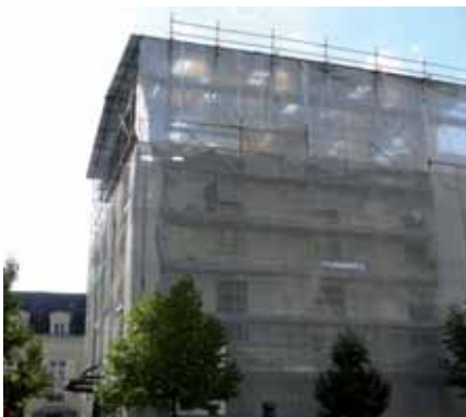
Renovation work on new building, Angers, France
