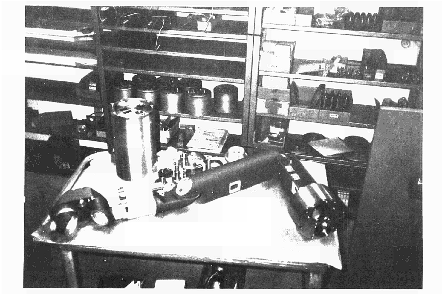
- FIGURE 3 - View of all segments of "ROLD" robot before assembling.
